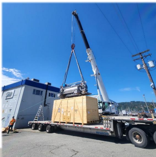
Unloading the HPP machine
