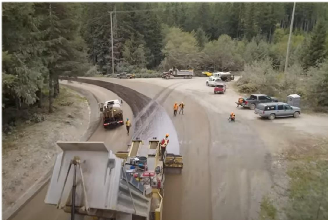
Work underway on the Bamfield Main
