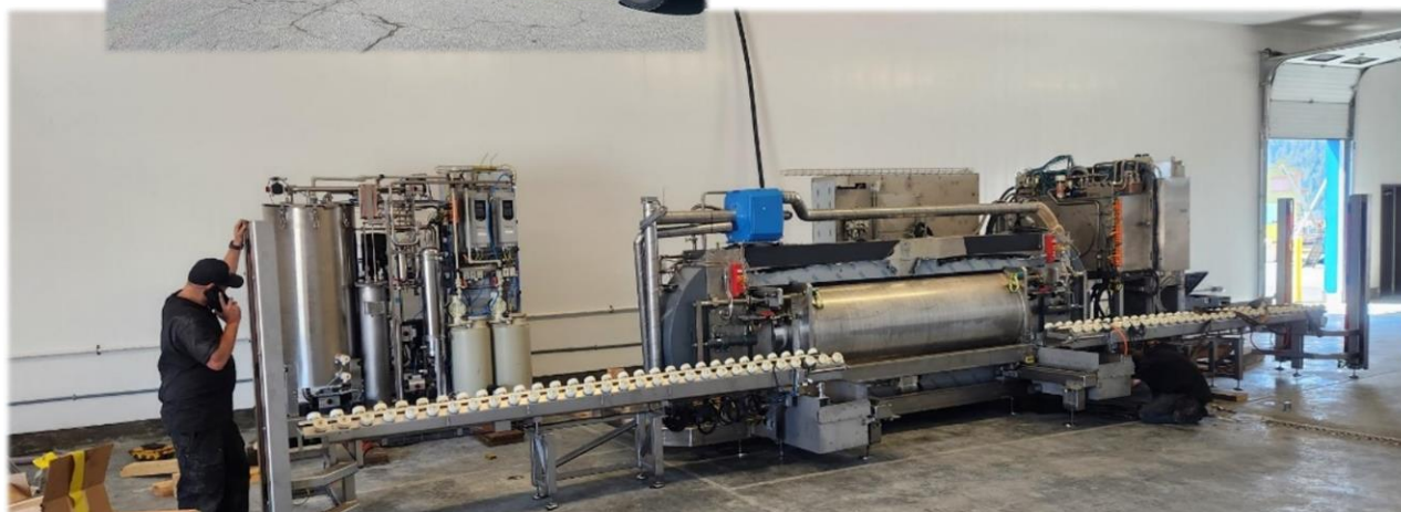
Assembling the HPP machine at the new Dock+ facility
